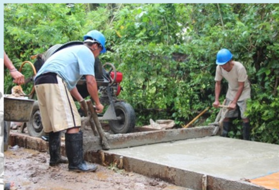
The laborers wearing their personal protective equipment during the construction of a concrete pathway in Brgy. Tigkiw, Gubat, Sorsogon.
